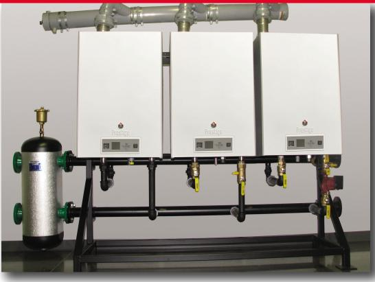
Note: Photo shows from left to right: Reverse Return, Reverse Return with Valves and Primary Secondary Piping Options. Hydronic Junction shown is included with Primary Secondary System only.
